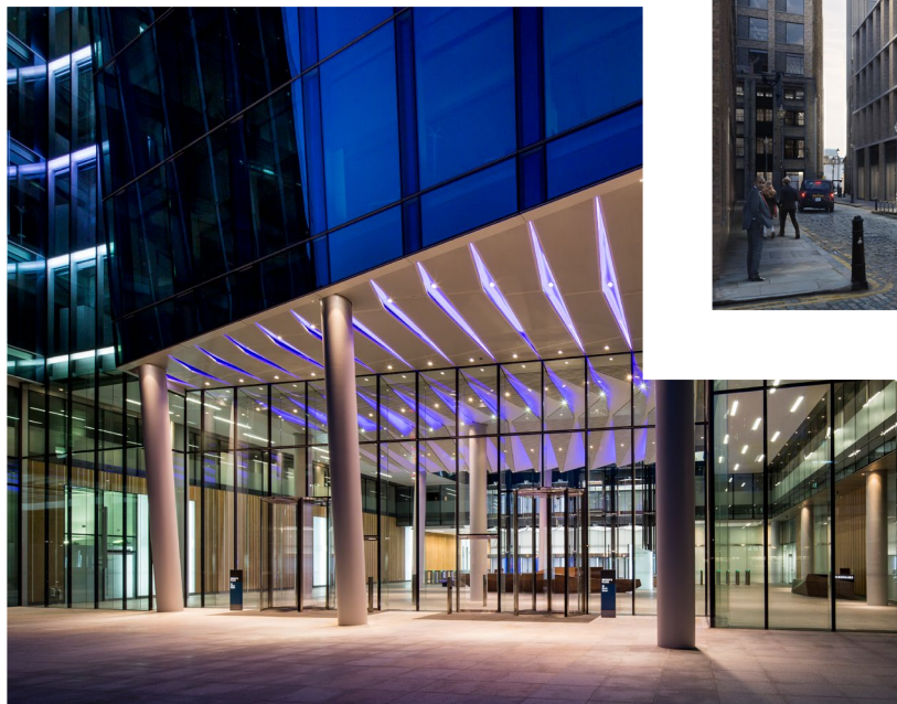
LED upgrades in back of house and selected public places at Regent's Place
