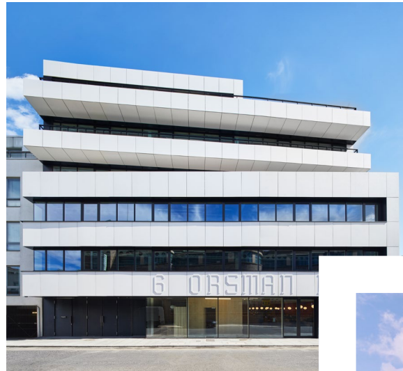
Orsman Road, Haggston, our first cross-laminated timber building
