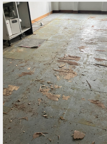
Example of damage that can be caused to raised access flooring from plywood being glued as a sub layer.
