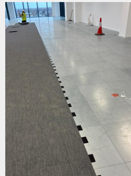
Midway through installation on the IOBAC MagTabs with the flooring contractor.
